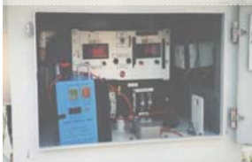
Current interrupter in circuit in T-R unit
